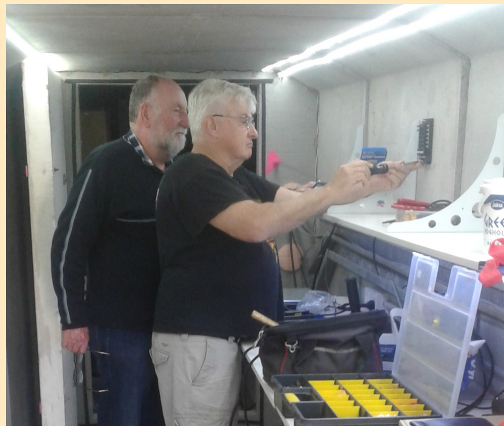
Paul & Blair fixing one of the fuse blocks in the control chamber.
