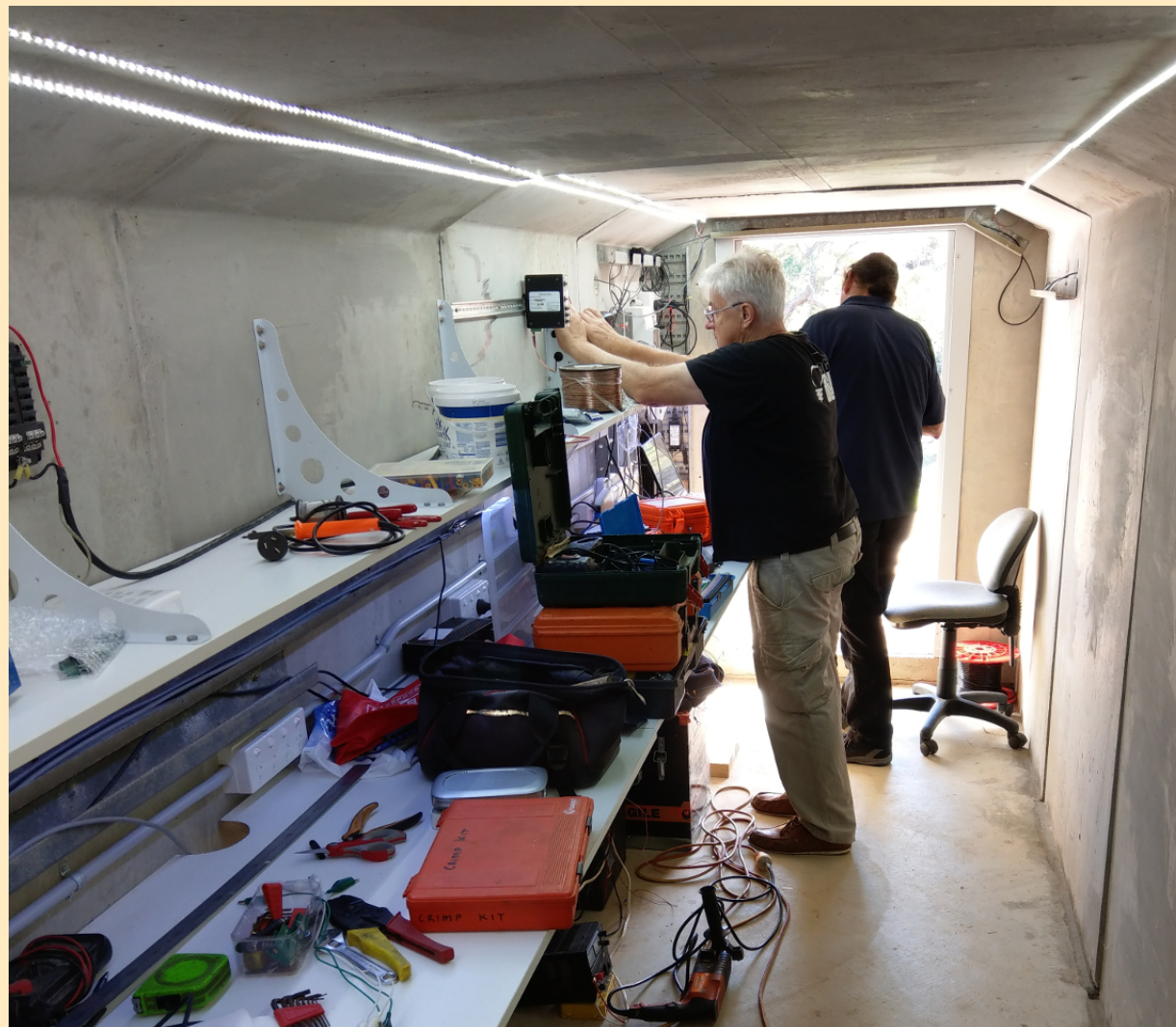
New cables and ring terminals, new network switch, new fuse blocks and fuses. Blair and Peter install the primary wiring infrastructure as a first step in the upgrade.
