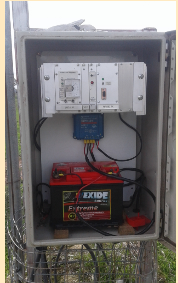
Inside the electronics box, the original equipment (inc. controller) the MPPT is above the battery.
