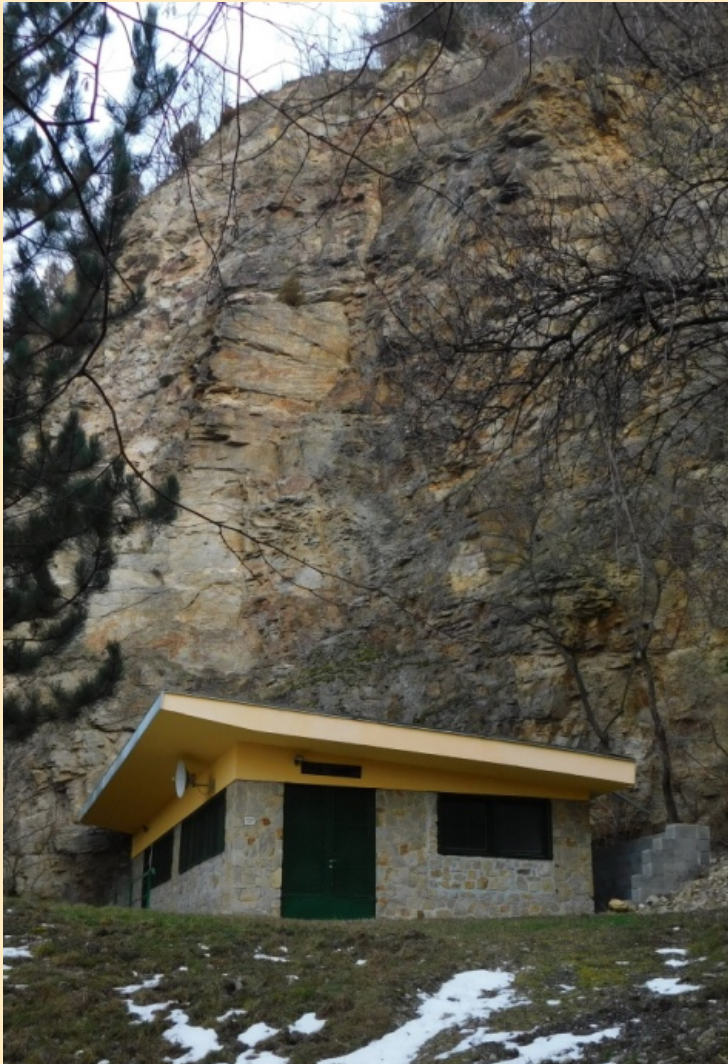
Figure 2: The entrance building of SOPGO under the 25 m high gneiss cliff
