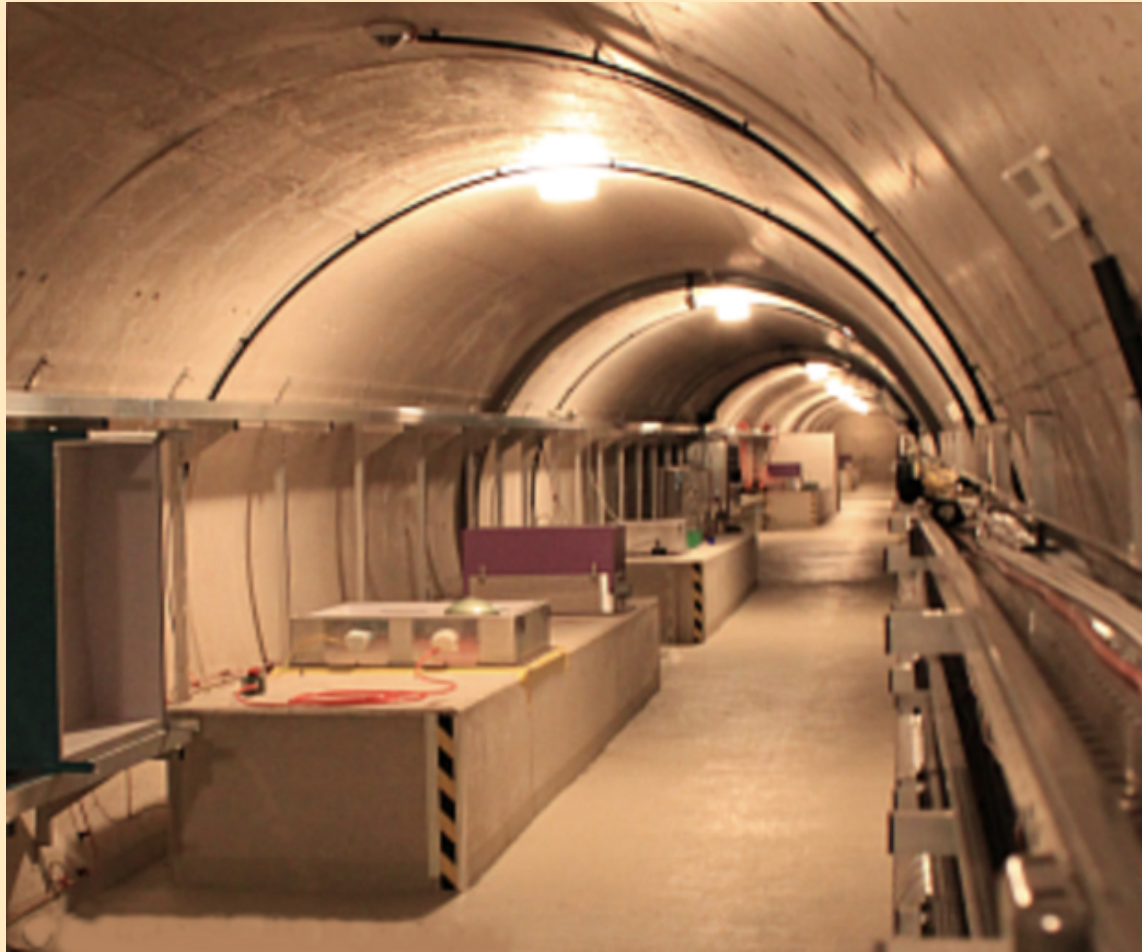
Figure 4: Instrument piers in the Conrad Observatoy SGO tunnel
