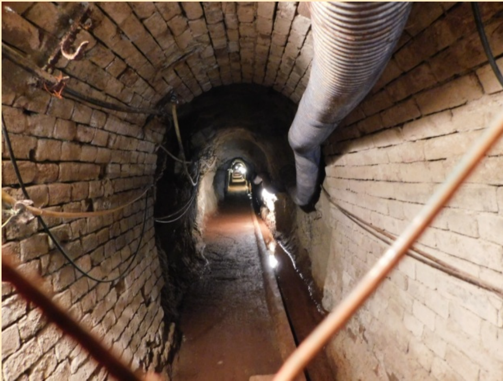
Figure 10: The main horizontal vault of Georgi Stollen
