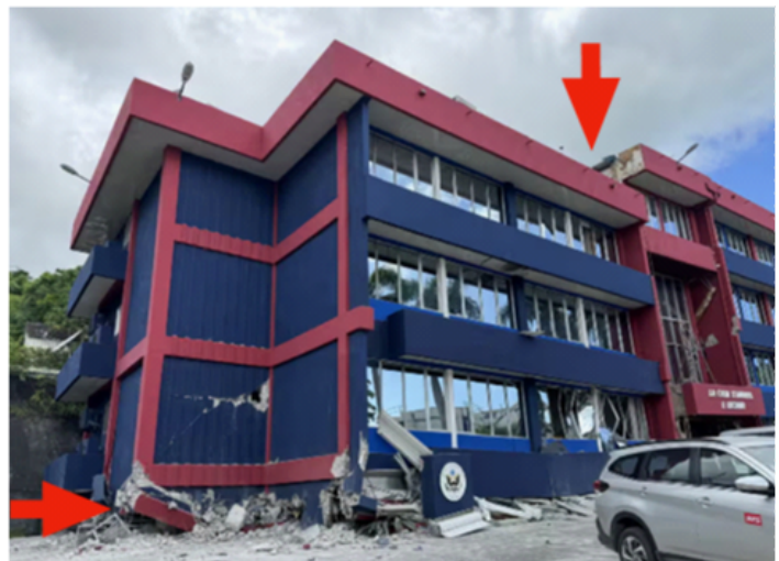
Photo 1: The building housing the American embassy and UK, French and NZ high commissions. At the time, many embassy staff had been outside the building having lunch. Note the missing ground floor level in the end section - arrows) as the storey collapsed.
