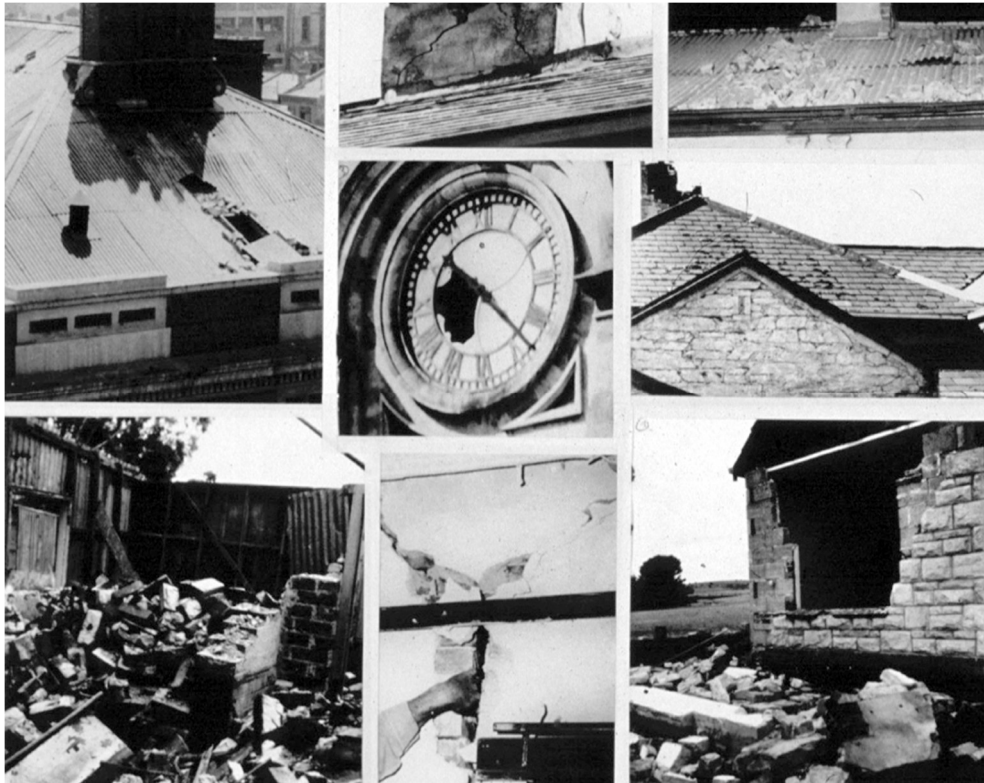
Figure 5 Photos of damage in Adelaide taken soon after the earthquake. The widespread use of unreinforced masonry, and damage, are very like that in Newcastle NSW following the M5.6 earthquake there in December 1989. In Newcastle many different assessors judged the maximum intensity at MMVIII and likewise in Adelaide. (McCue 2024)
