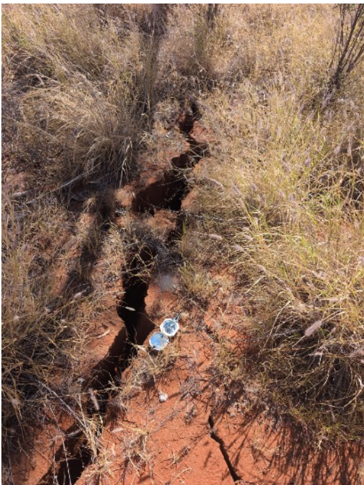
Photo The research team saw extensional cracking from the earthquake "stretching" the land surface. (Supplied: Quinn McNab). Shortly after, University of Melbourne researchers attended the scene and were met by a several-kilometre-long rupture in the ground.
